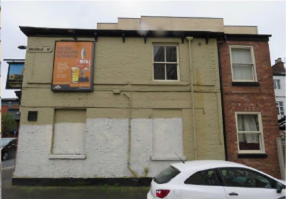
(Side Elevation from Brindle Street)
